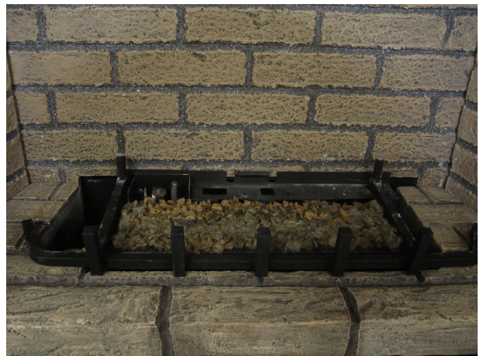
Figure 54 - Rock wool placement
