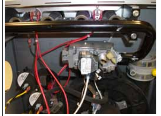
FIGURE 27 - INSHOT BURNER ASSEMBLY
