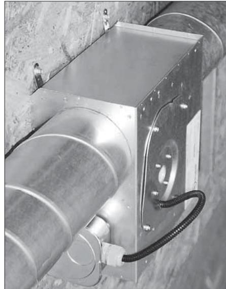
The 'LPK'-fan can easily be mounted with the four brackets in any position.
