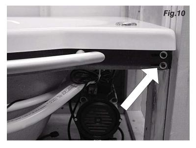
10. Towel Bar and Apron Panel are now fully installed. If necessary, apron panel may be removed by grasping the at the bottom edge between the kickbase and the panel and pulling outward. While holding, allow apron panel edge to drop free from under bath deck. Reassemble as directed in steps 9 and 10.
