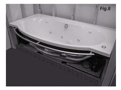
9. After adhesive has had appropriate time to cure, remove protective backing from the (4) tabs located on the rear bottom of the apron panel. Be careful that adhesive tabs do not contact dirt, dust, etc. Center the slots on the apron panel with the standoffs on the towel bar and slide the top edge of the panel between the deck edge of the bath and the towel bar support beam. Be sure that stepped edge of the bath. See Fig.13.
