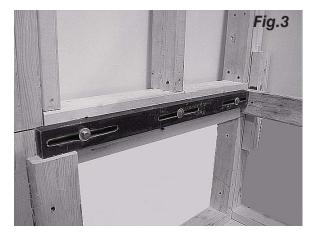
2. After installing back wall stringer, scribe a level plumb line at both ends of the recess opening. The line should extend from the top edge of the back wall stringer to the front of the recess opening. These lines will be used to locate the two end wall support stringers provided with the towel bar and apron kit. **See Fig. 2.**
