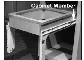
**Step 6:** Install wood unit (with slides attached) into cabinet, engaging product member slides into cabinet member slides push unit until it locks in place.
