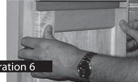
**Step 7:** Be sure bumper pads (not provided) are installed to all four corners of door. Push door closed and apply pressure to all four corners making sure door is flush with cabinet. (See illustration 6)
