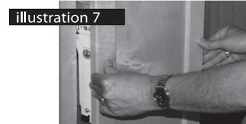
**Step 8:** Pull door open from sides of door at slide level. (See illustration 7). Make sure to securely tighten top screws.
