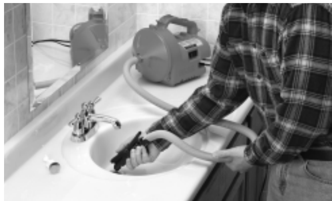
Figure 7 – Feeding Cable into Drain Opening
