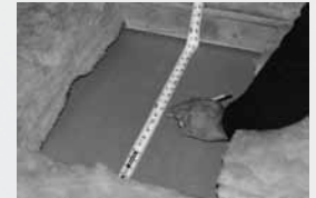
Inside attic fig. 2
