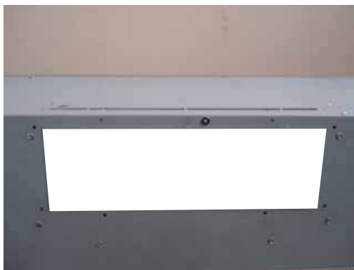
Horizontal Ducting (3-1/4"x10" Rectangular)
