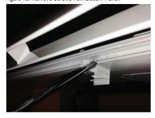
Figure 14: Latch over Screws on Indoor Unit Bottom Panel.
