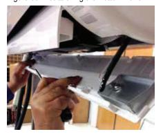
Figure 90: Reattaching the Screws on the Bottom Panel.
