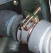
Figure 50: HVT and HSV5 Outdoor Unit Drain Hose Extension.
