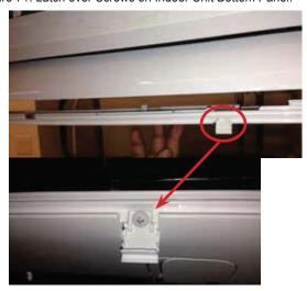
5. Remove the control cover on the bottom right side of the front of the indoor unit by detaching the screw. Set the screw and the control cover aside for re-installation.
