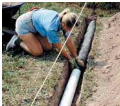
Figure 38: Underground Refrigerant Piping.
