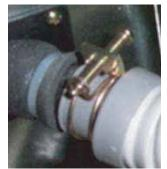
Clamp the Flexible Drain Hose Connection
