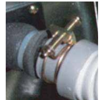
Clamp the Flexible Drain Hose Connection
