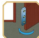
Pull door toward you to check if it's level. Observe contact of door to jam and make sure it's level. Adjust if necessary
