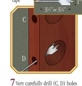
into door edge exactly at pencil marks. 3<sup>1</sup>/<sub>2</sub>" deep for a 2<sup>3</sup>/<sub>8</sub>" backset  $3\frac{1}{8}$ " deep for a  $2\frac{3}{4}$ " backset Helpful Hint: Mark edge depth of drilling with masking tape.
