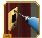
8 For Latch Strikeplate: Using latch strikeplate as a template, drill two <sup>1</sup>/<sub>8</sub>" pilot holes for the  $\#8 \times \frac{3}{4}$ " screws.
