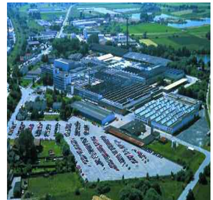
Stiebel Eltron's plant in Holzminden, Germany.
