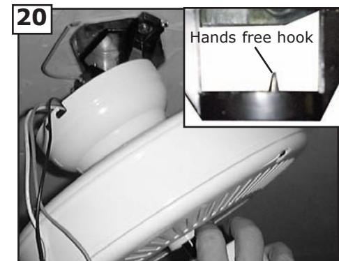
Hang fan from mounting bracket by the hands free hook into a closed hole on the edge of the Canopy.
