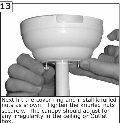
Next lift the cover ring and install knurled nuts as shown. Tighten the knurled nuts securely. The canopy should adjust for any irregularity in the ceiling or Outlet box.
