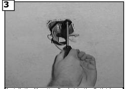
Install the Mounting Bracket to the Outlet box. Use only the screws provided with the outlet box.
