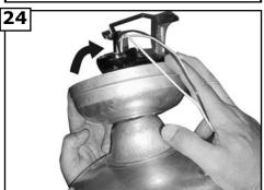
Use caution when hanging fan not to hold by blades are put any pressure on blades or blade arms. This could create problems of blade pitch deviation, deforming blade arms, or scratching of blades. Carefully lift fan assembly by fan body onto mounting bracket. Rotate fan so that the notch on the ball engages the ridge in the mounting bracket. This will allow hands-free wiring.
