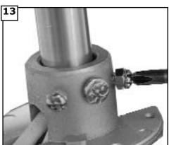
Tighten both yoke set screws to further secure downrod. Reinstall the downrod ball previously removed.
