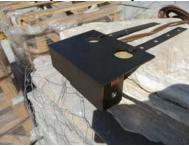
Weight of material stacked on top will hold unit in place. You can also use mortar, adhesive, and/or anchors.
