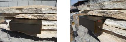
Stack stone, brick, or cap on top of straps and mortar plate to finish.
