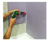
• Repeat this process on perpendicular tile also facing corner (image B). If corner trims are used, sealer should still be applied in trim channel.
