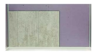
Apply adhesive to the back of the panel using Loctite® Power Grab Ultimate. Carefully read and follow
