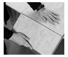
• Cut panels to accommodate shower heads and faucets. Measure and mark the borders where the opening will be with a marker. Drill a ½" to 1" hole using a drill in a corner of the cut-out section. Use a jigsaw or hole saw to cut the remaining opening, following your tracing.
