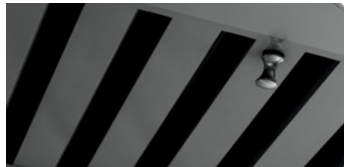
stainless steel baffle slot filters
