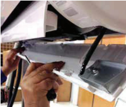
Figure 89: Reattaching the Bottom Panel.
