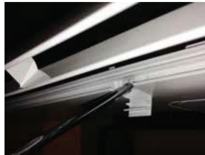
Figure 90: Reattaching the Screws on the Bottom Panel.
