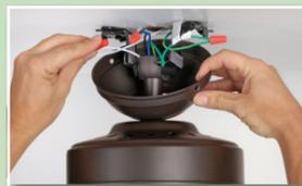
**2.** Attach to bracket and connect wires
